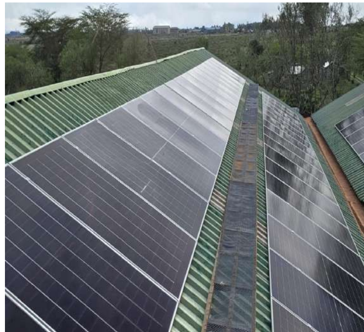
Ongoing 50kW Grid Tie Solar System installation at a Workshop in Kitengela Town, Kenya.
