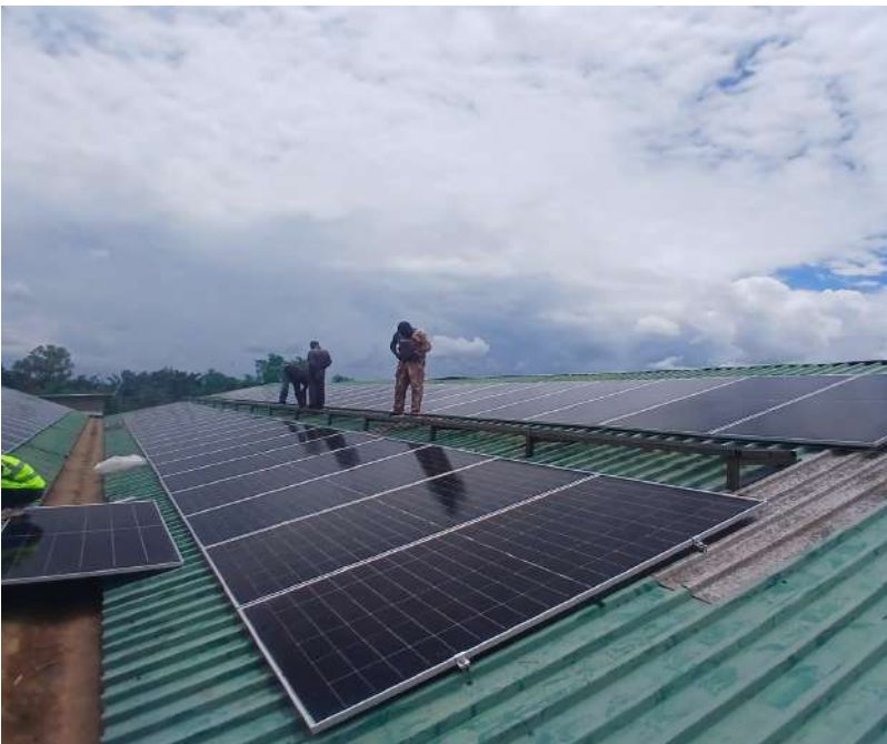
Ongoing 50kW Grid Tie Solar System installation at a Workshop in Kitengela Town, Kenya.
