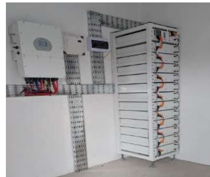
20kW with 61kWh battery storage project Successfully commissioned RDA at Chongwe district Zambia
