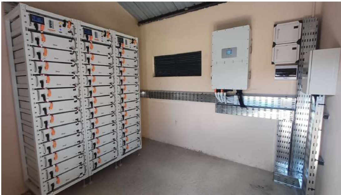
20kW with 61kWh battery storage project Successfully commissioned RDA at Chongwe district Zambia
