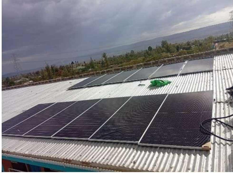
Luminous 11KVA Luminous Lithium Battery 10.24Kwh - 2pcs Jinko Solar panels 615W -12pcs Mike Apartment , Jogoo, Nakuru in Kenya.
