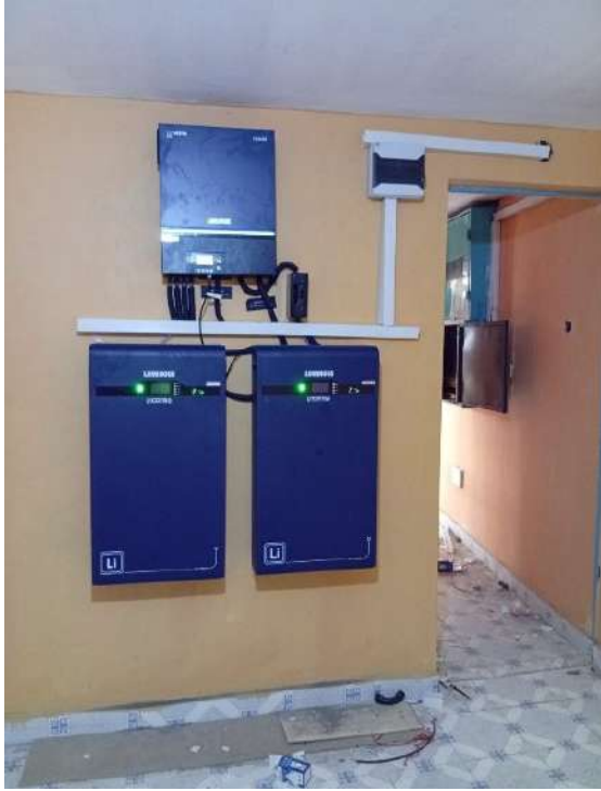
Luminous 11KVA Luminous Lithium Battery 10.24Kwh - 2pcs Jinko Solar panels 615W -12pcs Mike Apartment , Jogoo, Nakuru in Kenya.
